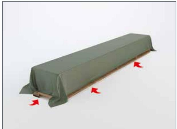
Store materials under a dry and well-ventilated tarpaulin. If the product becomes damp, it should be placed on its vertical edge to allow rapid drying. Never install wet products.
