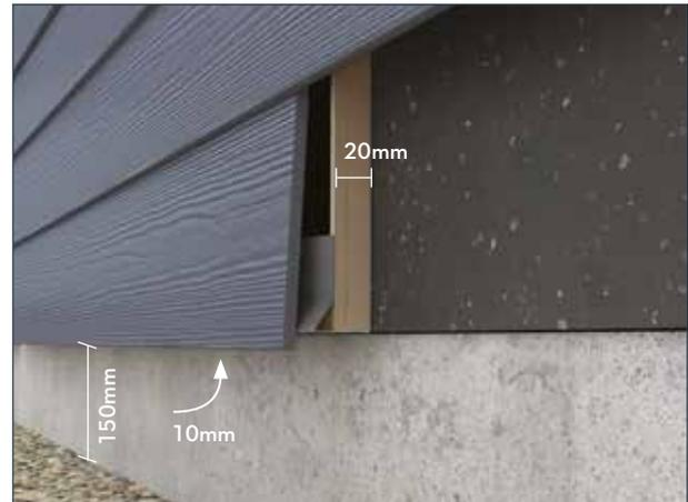
There must be a minimum of 5mm (vertical) and 10mm (horizontal) clearance around windows/doors-/framing/metal trim and other building materials to allow for structural movements and proper water drainage and ventilation.
