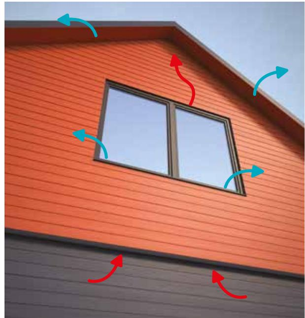
This passage must be a minimum of 10mm in the top and bottom or equal 100mm per m<sup>2</sup>. If grids or similar are used, the openings must equal 100cm<sup>2</sup> per linear meter.
